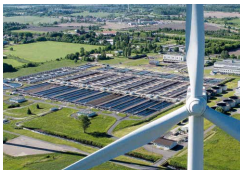
Schönerlinde sewage treatment plant is heading for energy self-sufficiency. © Berliner Wasserbetriebe
